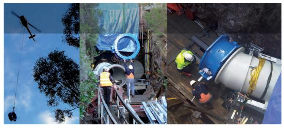
One of the old butterfly valves was also planned for renewal during the refurbishment. VAG-Armaturen in Germany quickly found the perfect fit: a VAG EKN Butterfly Valve, DN 1200, PN 16 with manual hydraulic drive.
