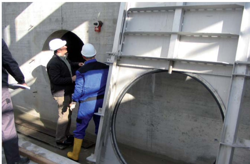
For the supply and draining of cooling water to and from the tower, VAG recommended VAG EROX® Sluice Gate Valves because they are particularly reliable and have a tight seal.
