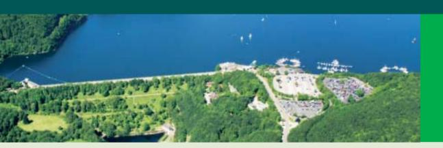
The Rur dam Schwammenauel in the North Eifel mountains has a capacity of 203 million m³, making it one of Germany's largest dams. It catches the rainfall in the headwaters of the Rur. The Schwammenauel power station uses the hydropower station to generate electricity.
