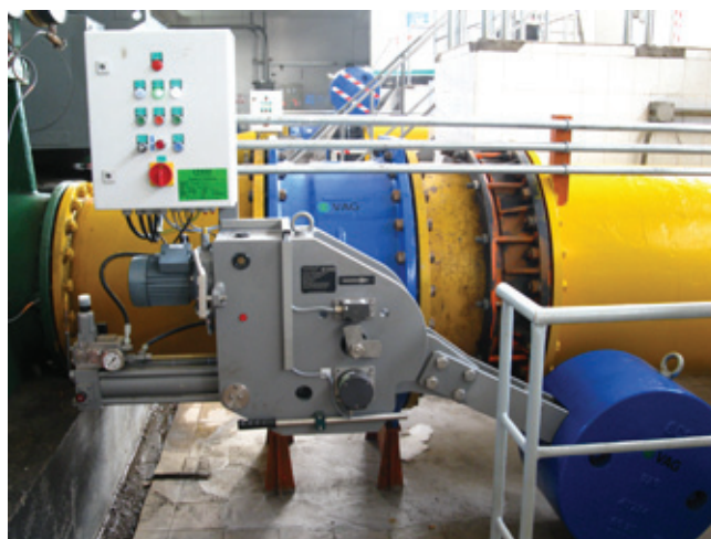
VAG EKN® Butterfly Valve + VAG HYsec hydraulic brake and lift unit
