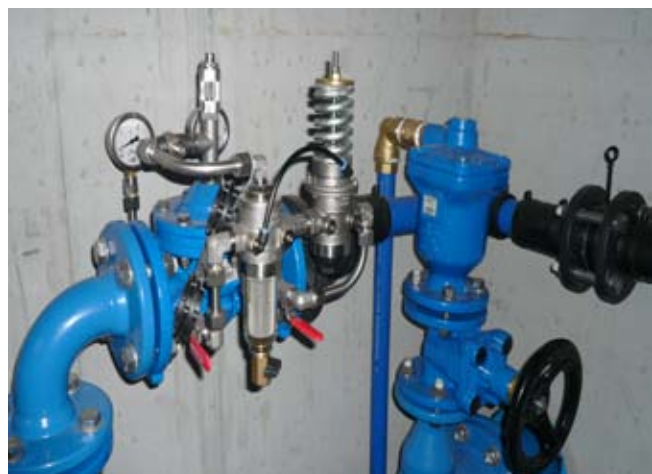
A VAG PICO® Control Valve as a safety valve with VAG BEV Venting Equipment
