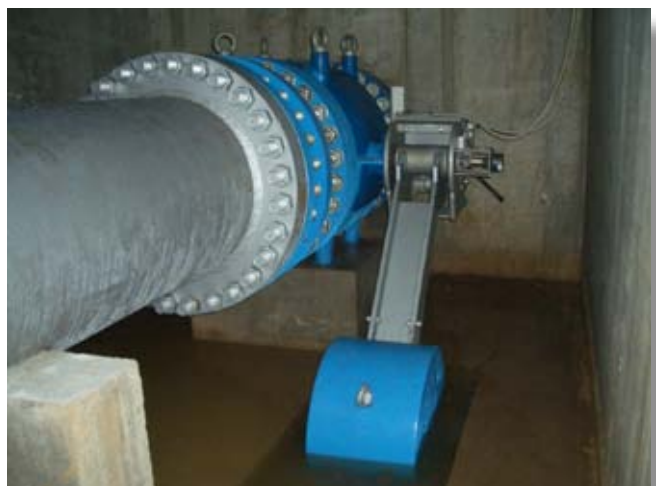
VAG RIKO® Plunger Valve with hydraulic brake and lift unit DN 600 PN 100
