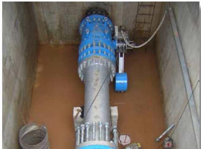
Water supply pipeline equipped with a VAG RIKO® Plunger Valve with hydraulic brake and lift unit
