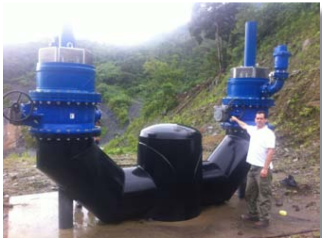
VAG EKN® Butterfly Valve DN 800 with VAG Spring Loaded Air Valves DN 800
