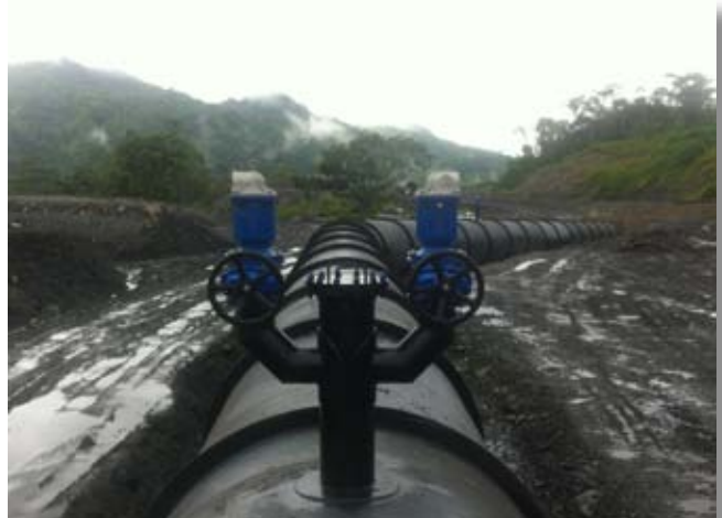
VAG DUOJET® Automatic Air Valves DN 200 and VAG EKO® plus Gate Valve DN 200
