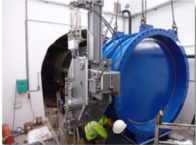
Installation of the operational valve in the structure
