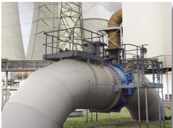
VAG EKN® Butterfly Valve with double-sided UWV safety interlock as unit isolation valve DN 2000
