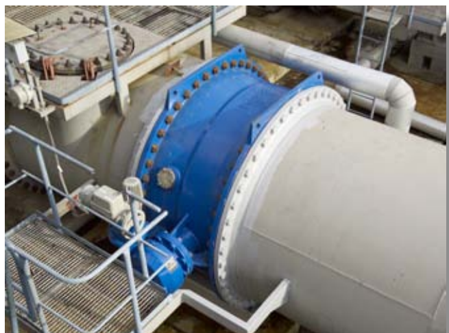
VAG EKN® Butterfly Valve with one-sided UVV safety interlock
