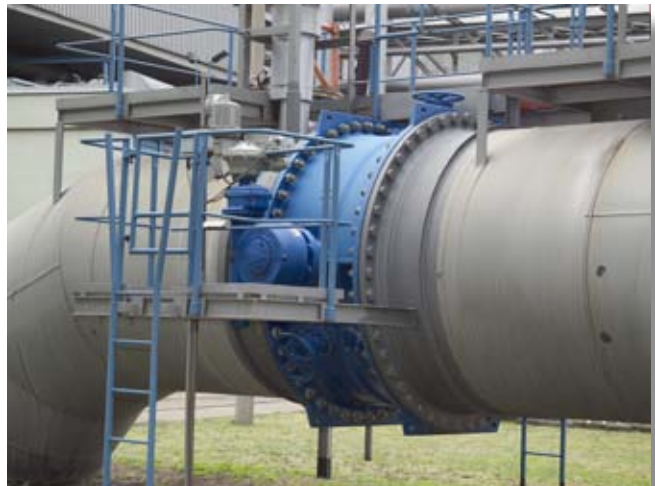
VAG EKN® Butterfly Valve with double-sided UVV safety interlock as unit isolation valve DN 2000
