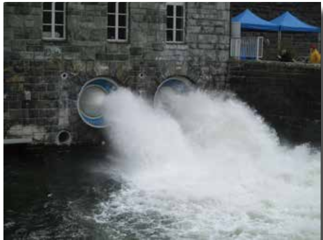
The new bottom outlet valves in operation
