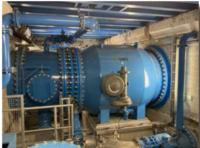
Installed VAG RIKO® Plunger Valve DN 2000
