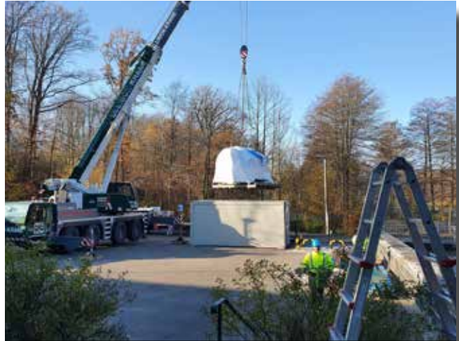
Due to a special design, the weight of the valve could be reduced to 15 tons.
