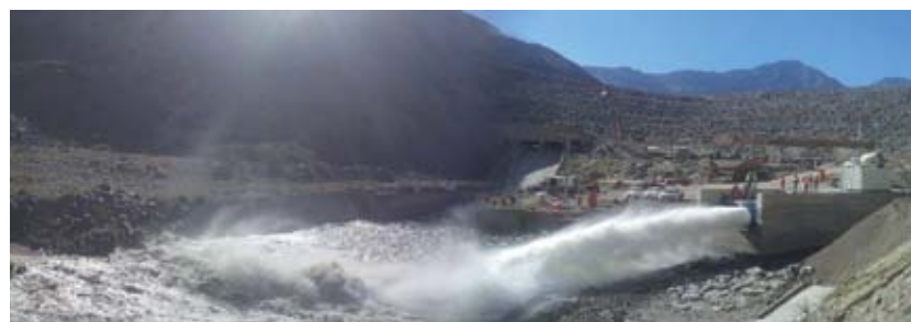
VAG KSS Hollow-Jet Discharge Valves at the bottom outlet of the El Yeso Dam
