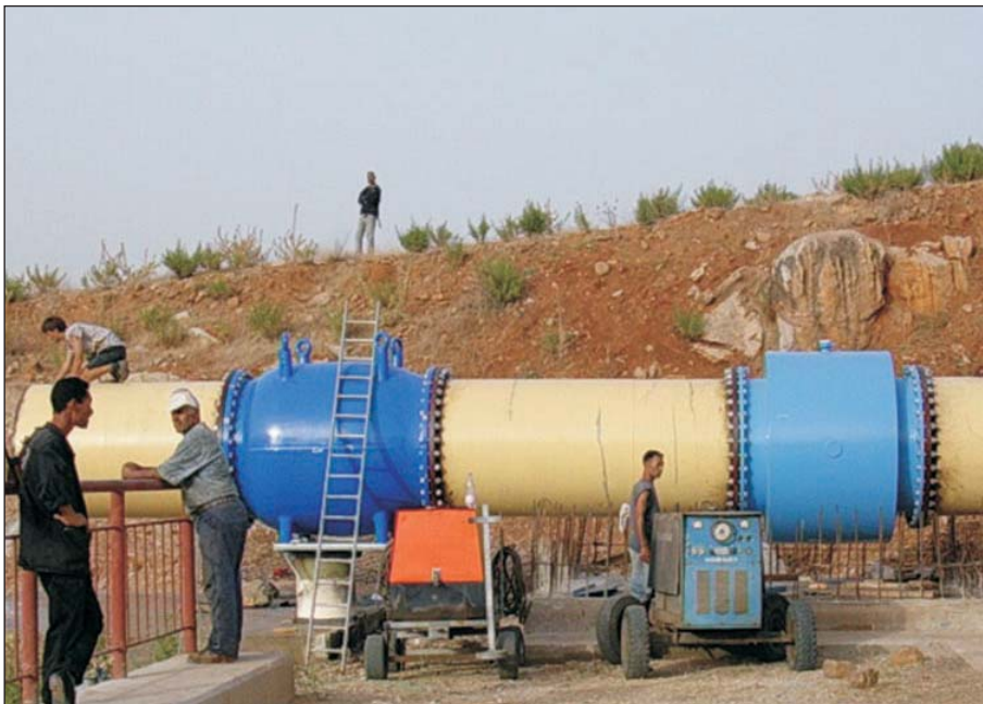
Fig. 7: VAG Plunger valve DN 800 including an inductive flow meter at SMBA dam, Algeria
