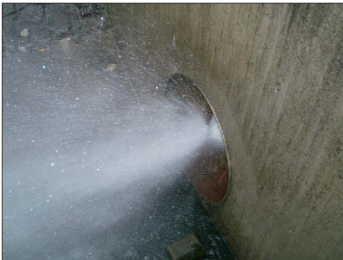
Fig. 3: Closing process of a VAG Plunger valve DN 800 installed in the bottom outlet of the Glör dam, Germany
