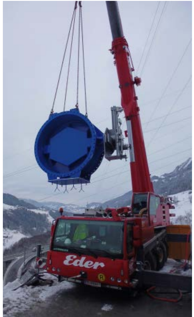
Picture: Large butterfly valve being transported to the site
