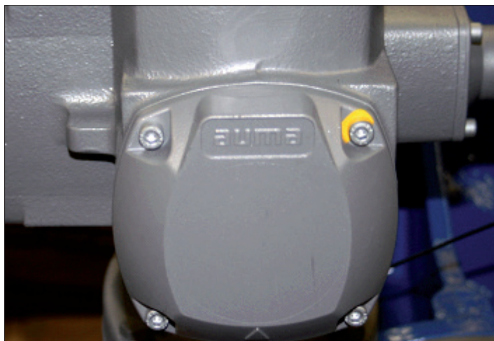
Picture 11: Secured bolts on the electric actuator
